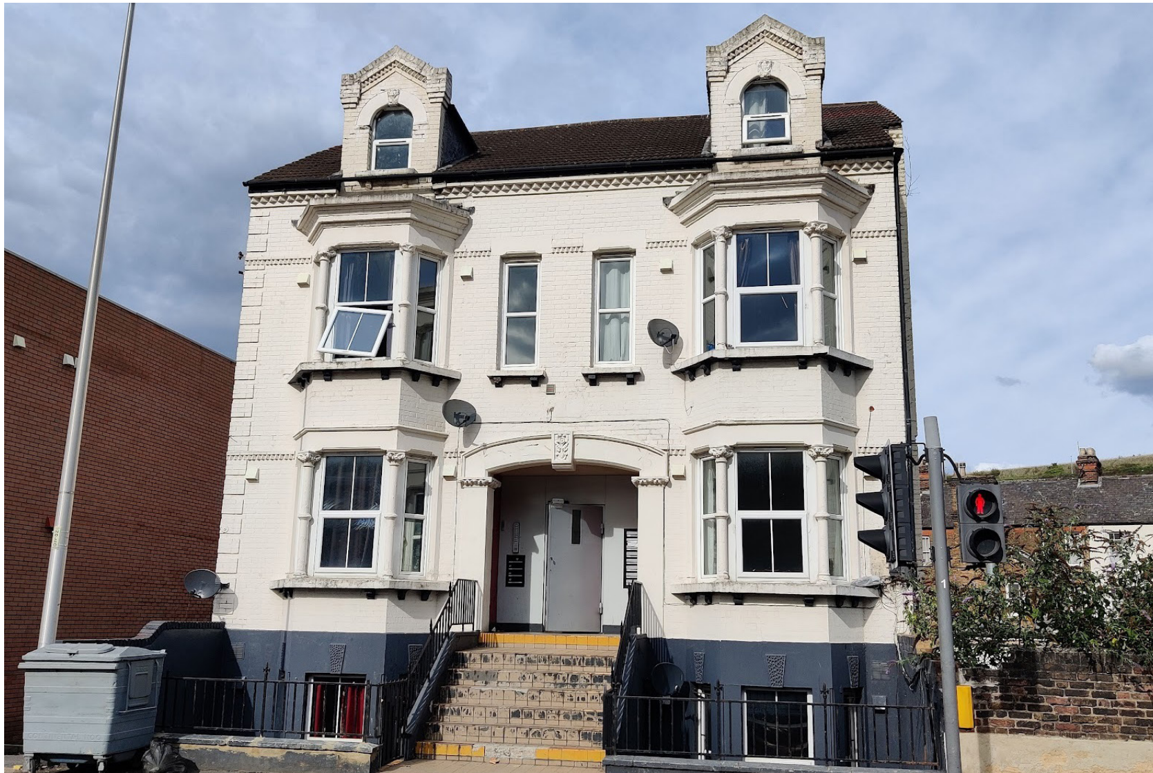
Figure 14 Loxley House, 219 New Road, Chatham
