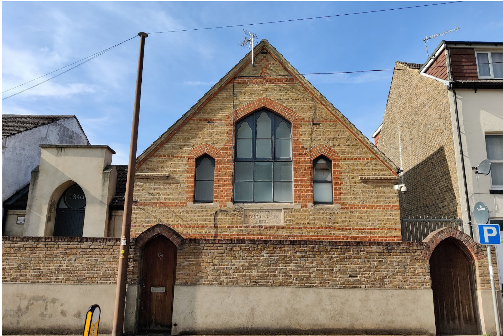
Figure 7 134a Luton Road, Chatham
