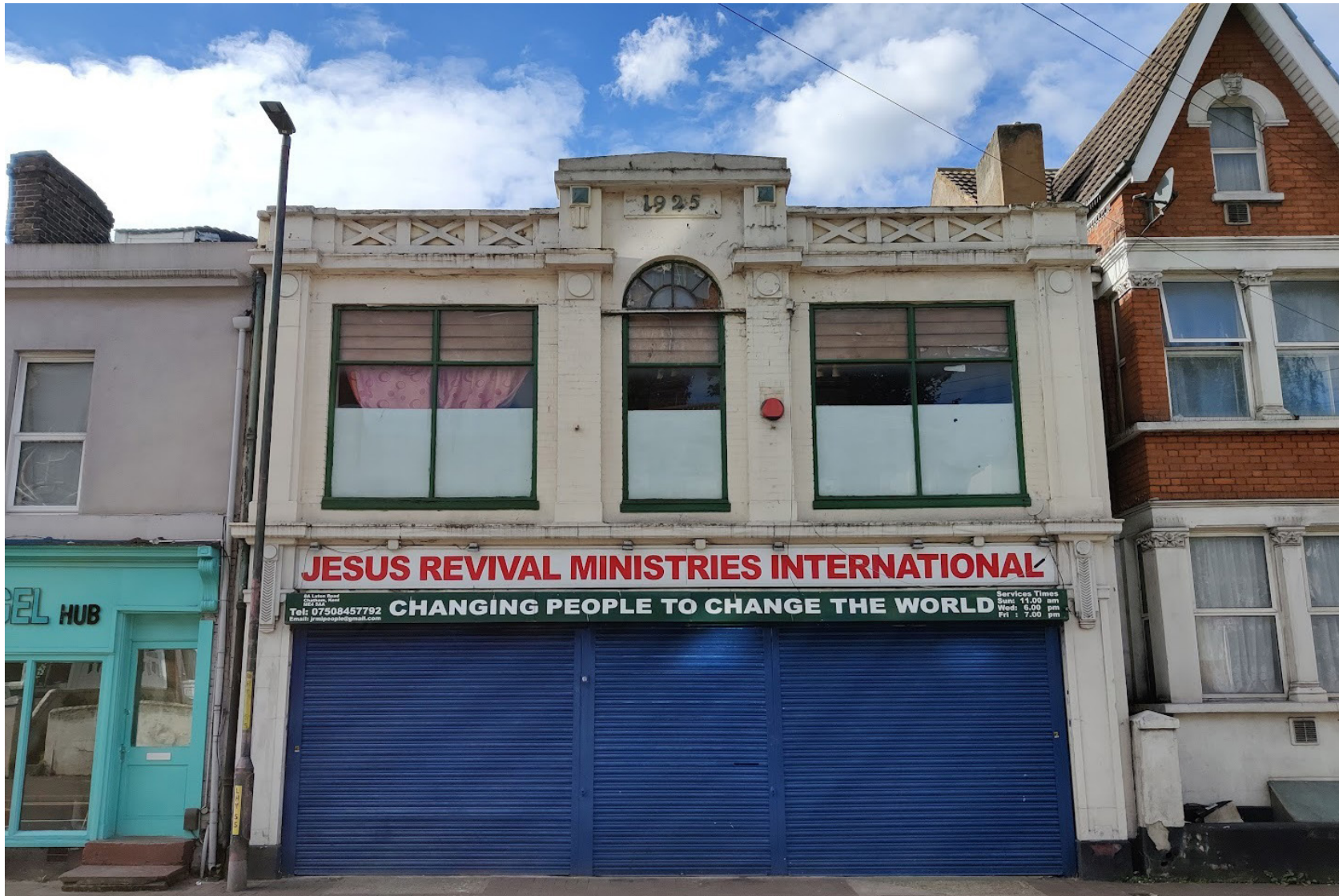
Figure 5 8a Luton Road, Chatham
