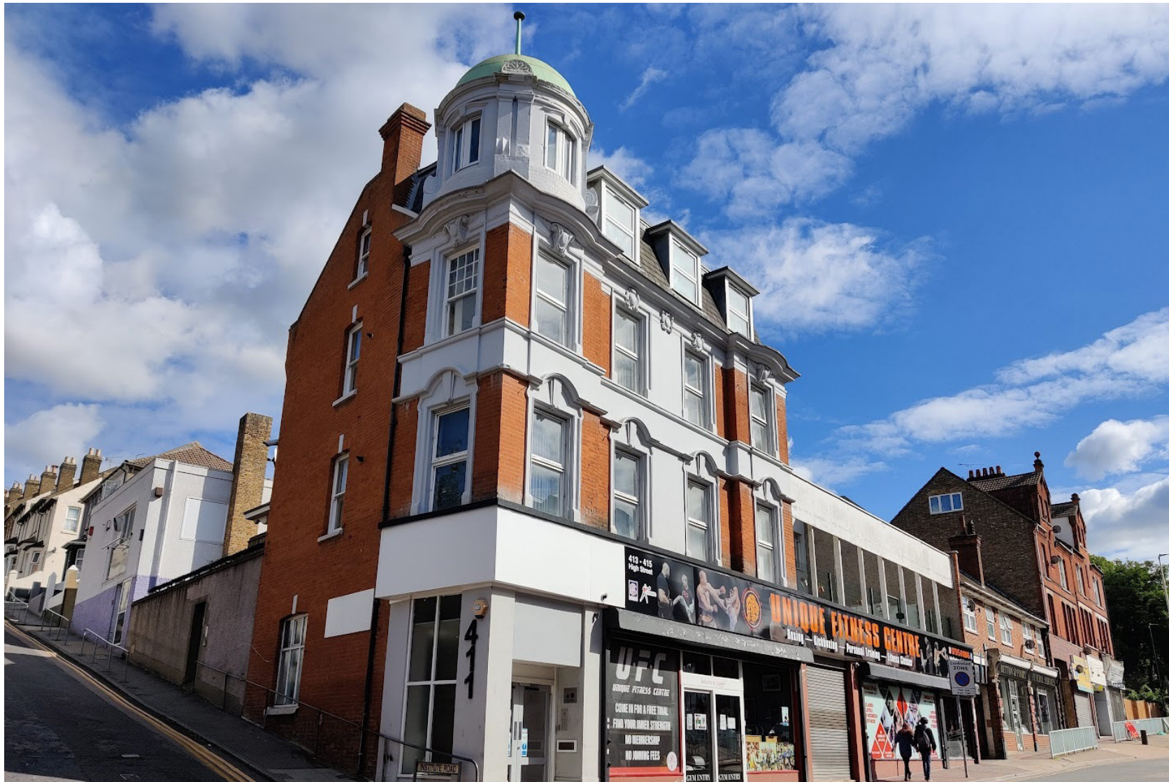
Figure 2 411 High Street, Chatham
