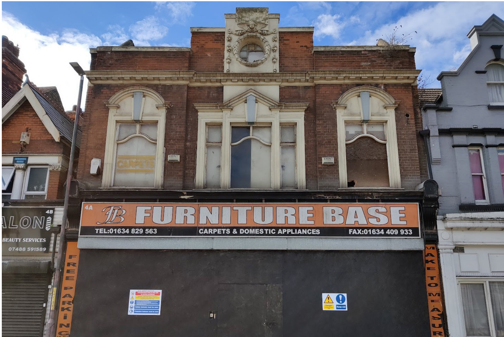
Figure 4 4a Luton Road, Chatham
